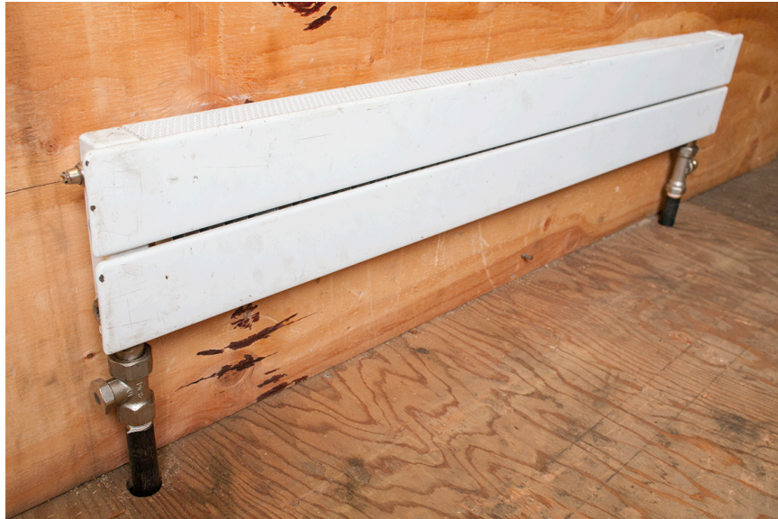
Figure 2 An installed panel radiator. (Skilled Trades BC, 2021) Used with permission.
