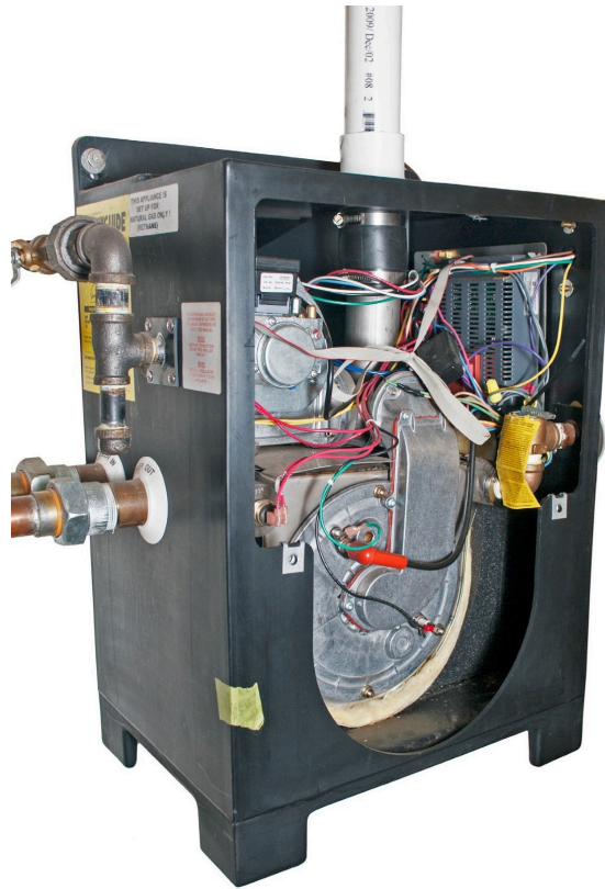
Figure 9 Condensing boiler. (Skilled Trades BC, 2021) Used with permission.
