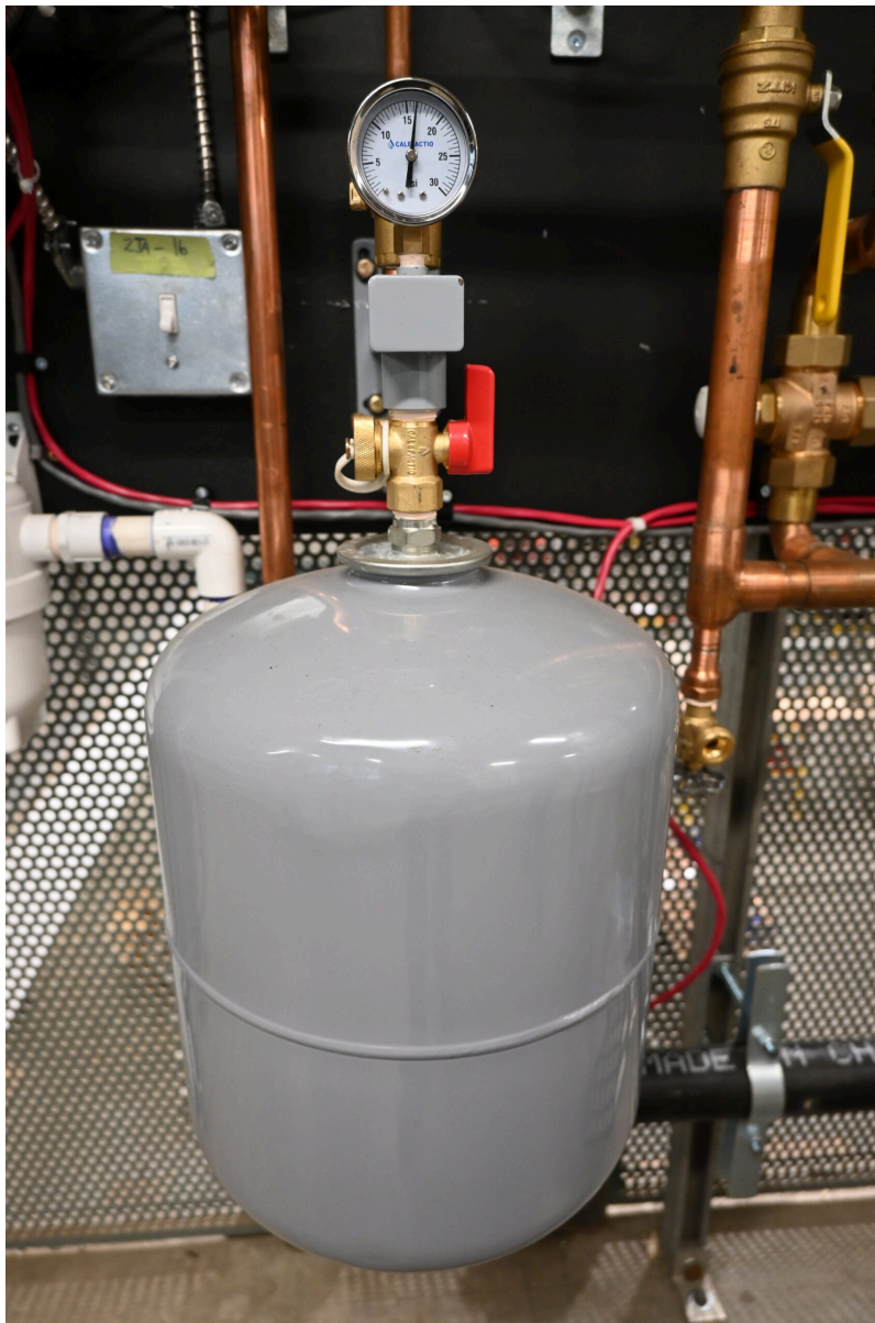
Hydronic expansion tank. (TRU Open Press) CC BY NC SA ( https://creativecommons.org/licenses/by-nc-sa/4.0/deed.en )
