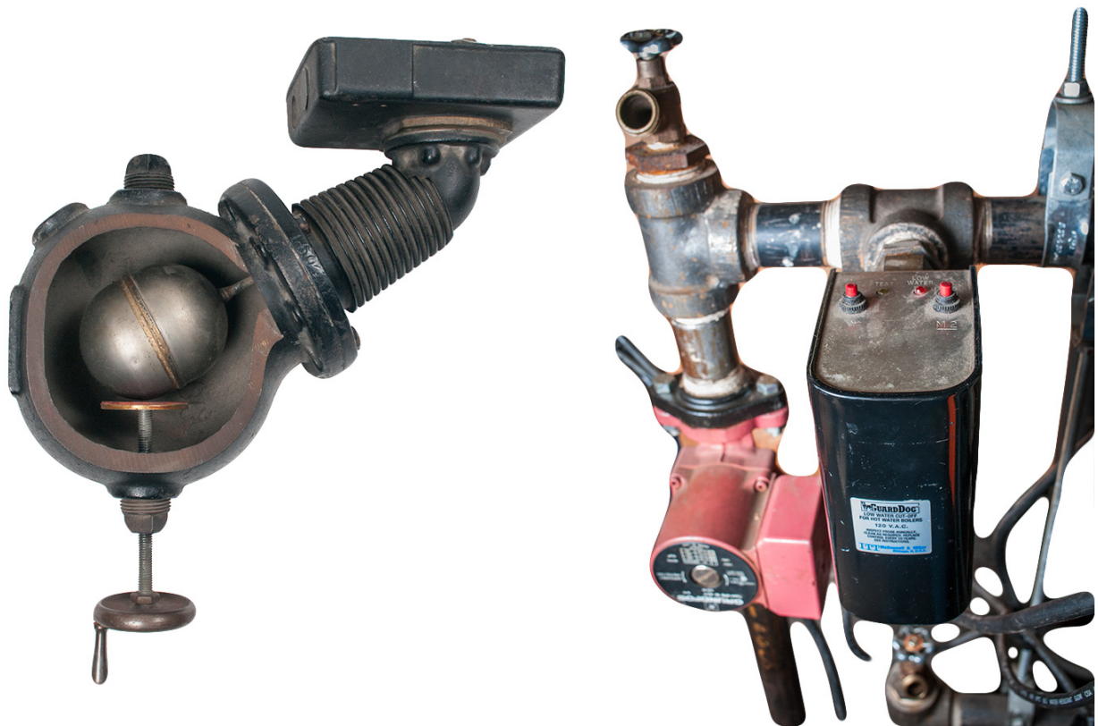
Figure 36 Float type low-water cutoff (left) & probe-type low-water cutoff (right). (Skilled Trades BC, 2021) Used with permission.
