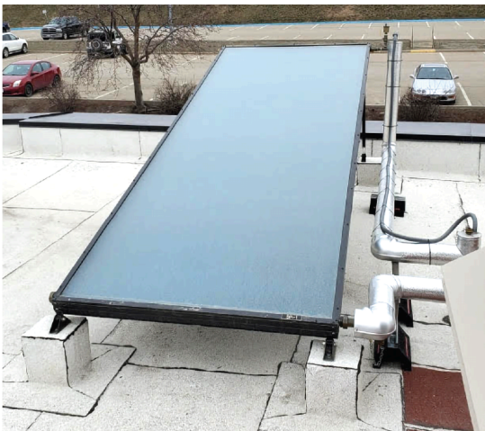
Figure 14 Flat-plate collectors. (Skilled Trades BC, 2021) Used with permission.
