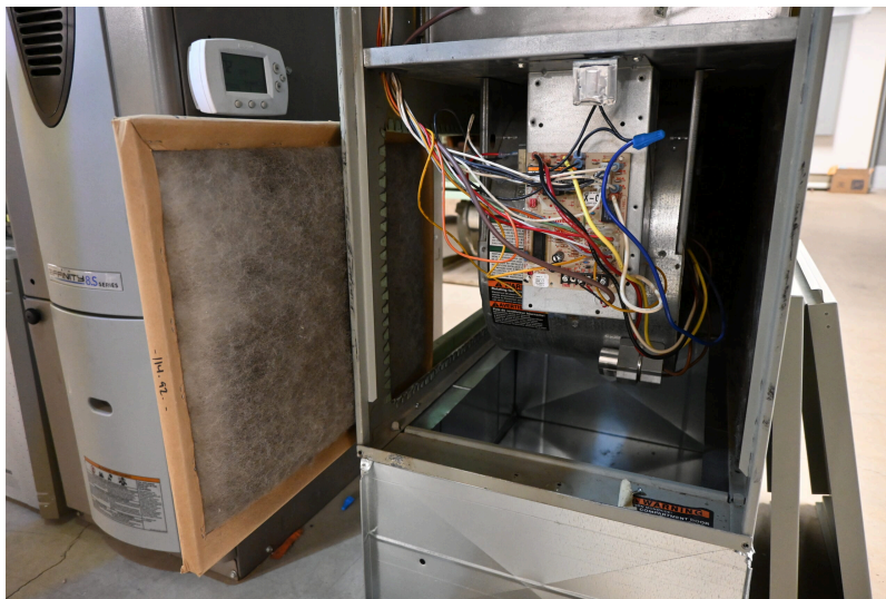
Figure 1 Forced air furnace media filter installation. (TRU Open Press) CC BY-NC-SA ( https://creativecommons.org/licenses/by-nc-sa/4.0/deed.en )
