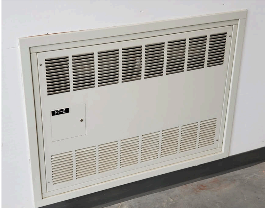
Figure 9 Forced-flow wall convector. (Skilled Trades BC, 2021) Used with permission.
