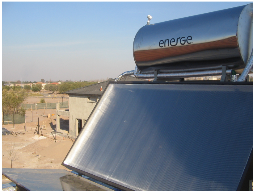
Figure 19 Thermosiphon system. (Skilled Trades BC, 2021) Used with permission.
