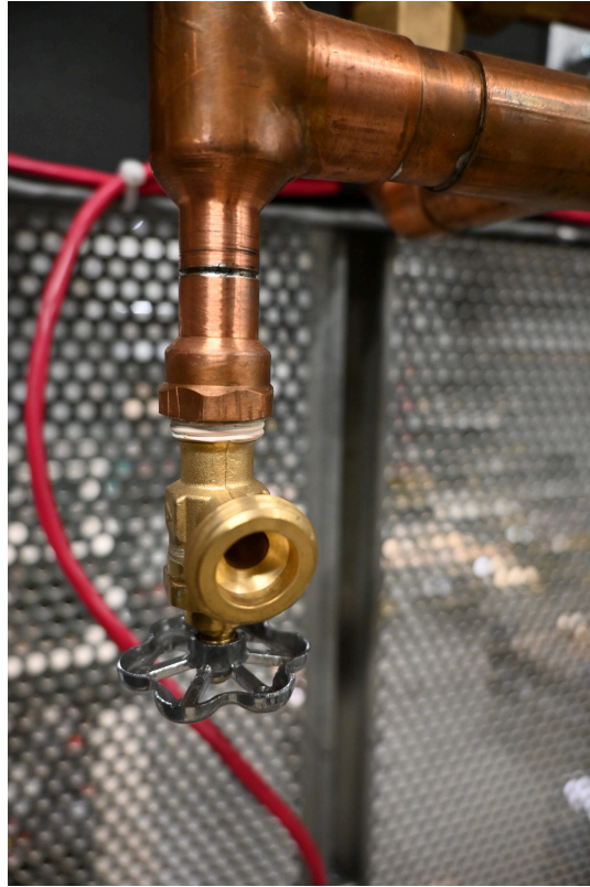
Figure 8 Purge valve/drain valve. (TRU Open Press) CC BY NC SA ( https://creativecommons.org/licenses/by-nc-sa/4.0/deed.en )
